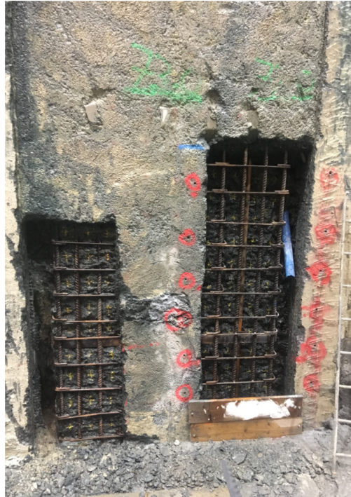
Infilled concrete at 71.5mATD
