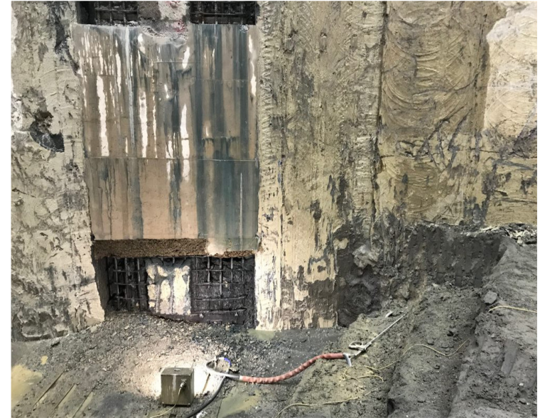
Repaired concrete at 69mATD
