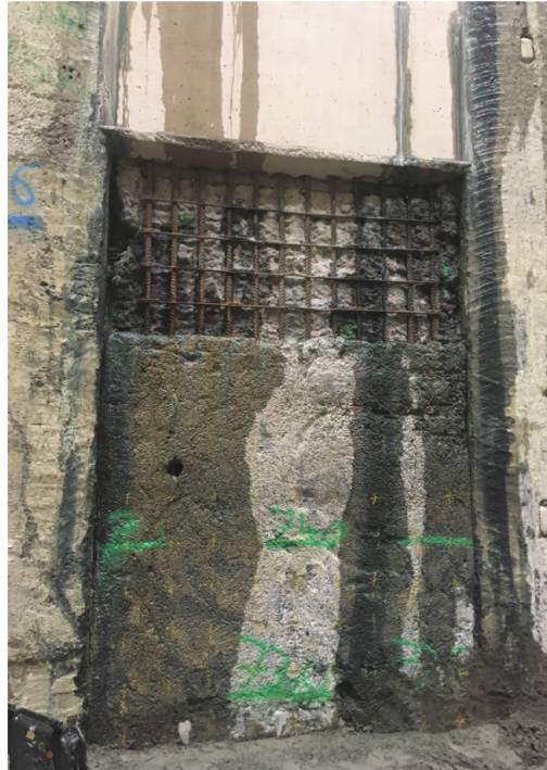
Infilled concrete at 73mATD
