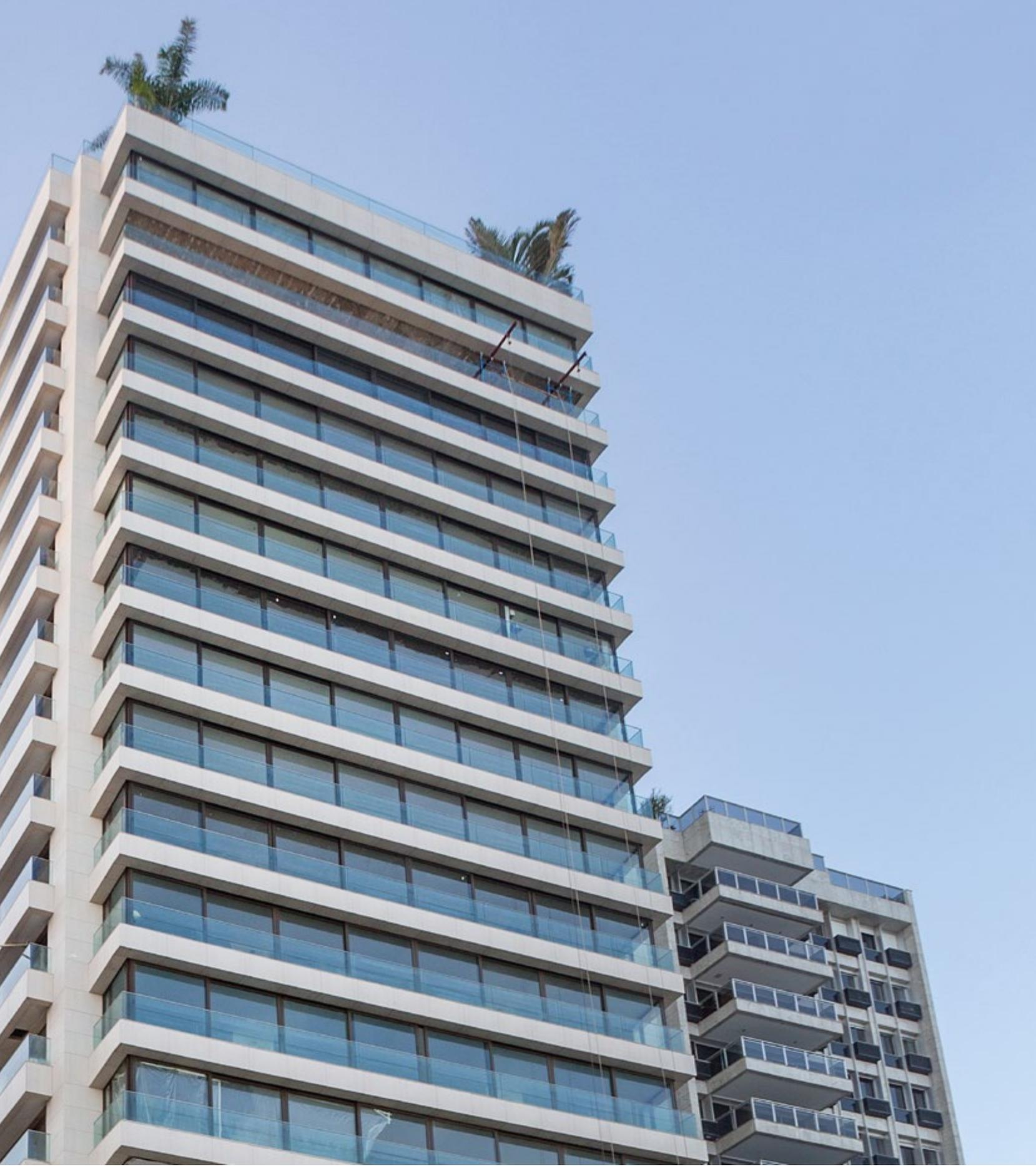
The biggest challenge faced by the project team was to find a new cladding that could be installed over the original material and would entail a maximum load of 90 kilograms per square metre. In addition, due to the building's proximity to the sea, the chosen material needed to match the exterior aesthetic with a subtle tone that blended into the surroundings as well as having mechanical properties to withstand the environmental damage that is common to such locations.
