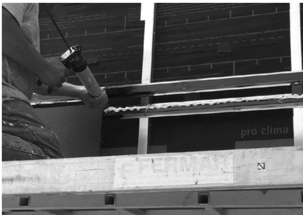
Fixing with chemical anchoring on profiles.
