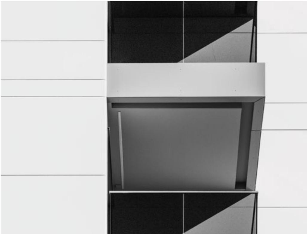
Hidden mechanical fixing with metallic profile on the continuous groove of the edge of the piece.
