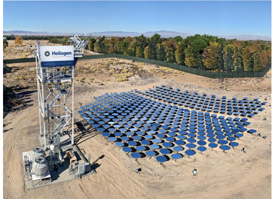
Heliogen's demonstration facility in Lancaster, California
