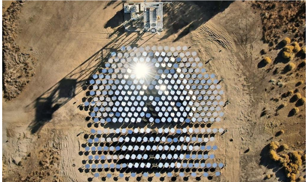
Heliogen's demonstration facility in Lancaster, California
