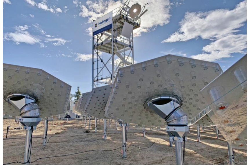
Heliogen's demonstration facility in Lancaster, California
