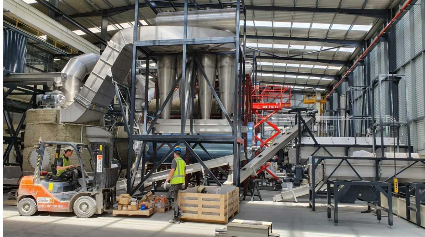
Construction-phase of 6 torrefaction lines (Futerra, Portugal)
