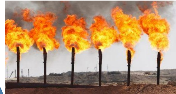
Significant amounts of flared gas, generating waste heat and emitting GHG
